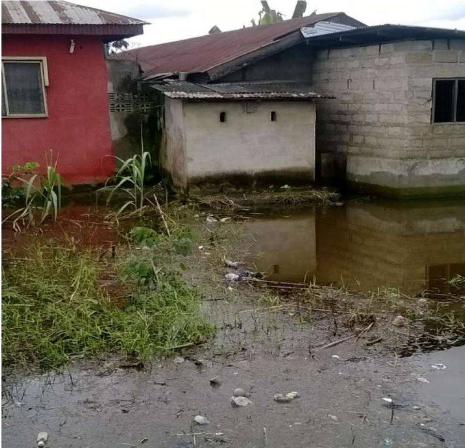
Figure 7: Abandoned Buildings During Flood in Mben Inyang Community. Source: Field Research (2018)
