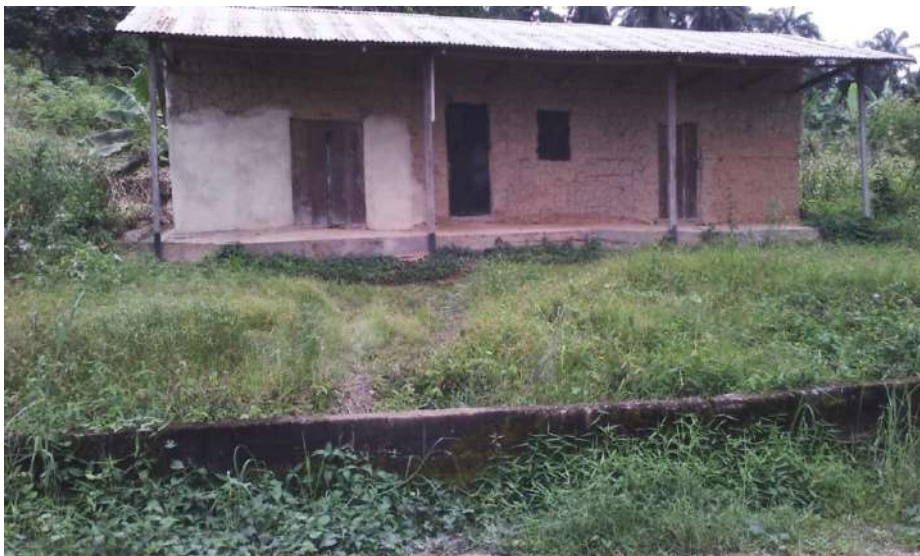
Figure 3: Barrier and Contour Constructed in Afia Isong Community to Restrict Flood Water Source: Field Research (2018)
