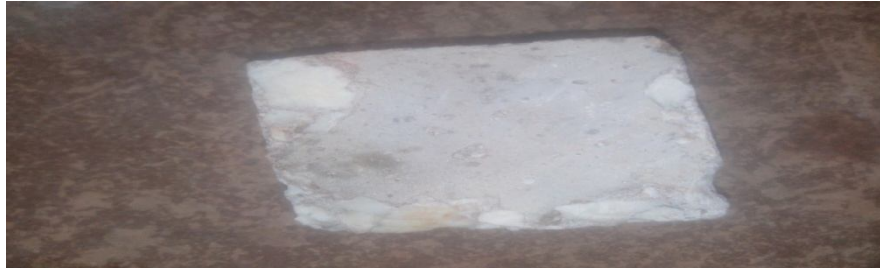
Plate II: Concrete cast with clam shell aggregates
