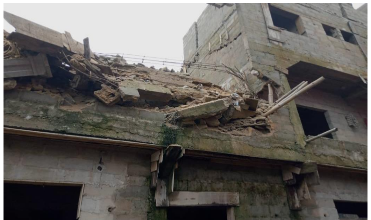
Fig 3: No 85 Azikiwe Street Aba. Collapse of three storey building under construction
